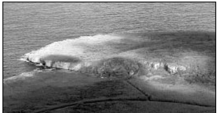
Photo 14: Aerial view showing the fault at Puntan Chiget, Tinian. Photo by John Mylroie.
